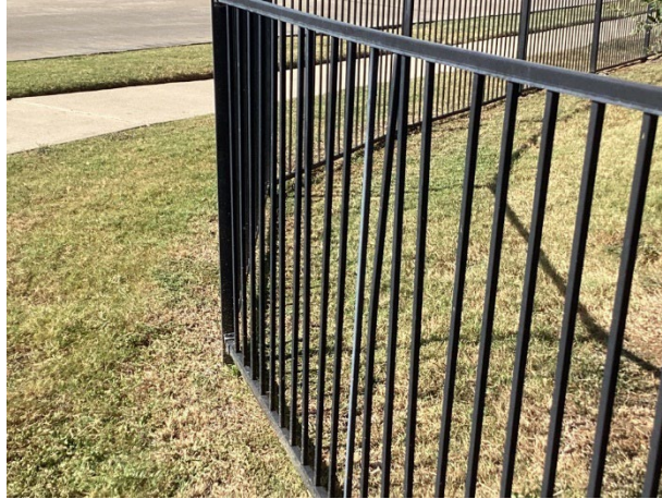
Fence picket damage at the splash pad
