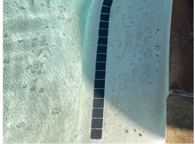
Plaster deterioration
