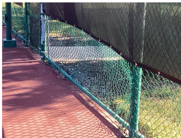
Fence warped webbing
