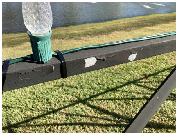
Fence finish deterioration
