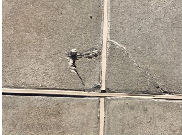
Concrete spalls
