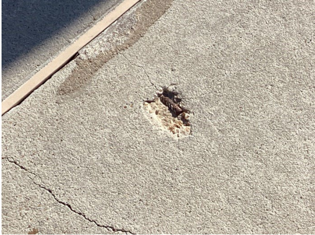
Concrete spalls and exposed reinforcement steel
