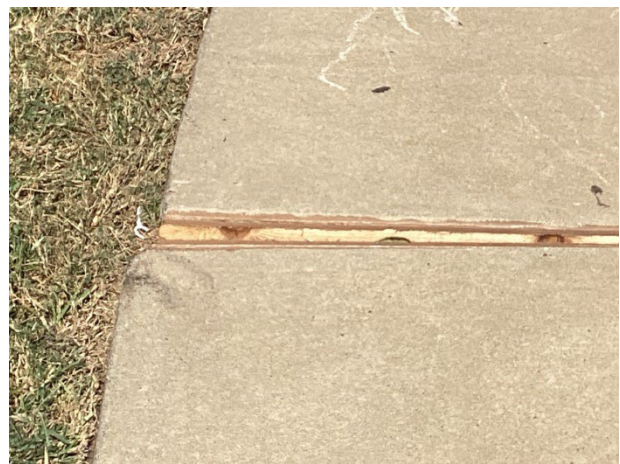
Sidewalk trip hazard
