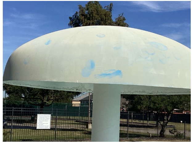
Finish deterioration
