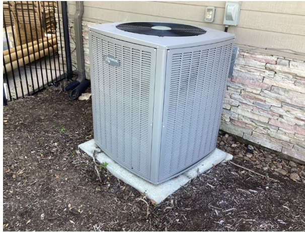
Split system condensing unit
