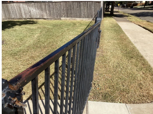
Fence leaning section at the splash pad
